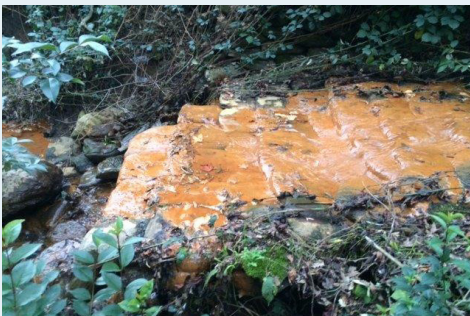
Iron-oxidizing bacteria growing on concrete just downstream of a storm drain outfall. Photographer Bené da Silva.
