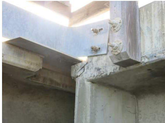
Photograph 18: Expansion joint - south side
