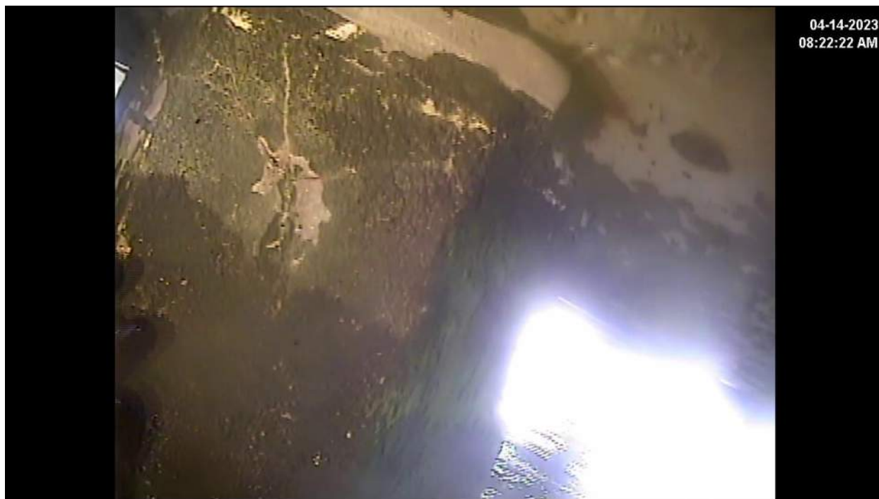
Photo 6 – C14 – Diver notes moderate cracking around the top of the pile.
