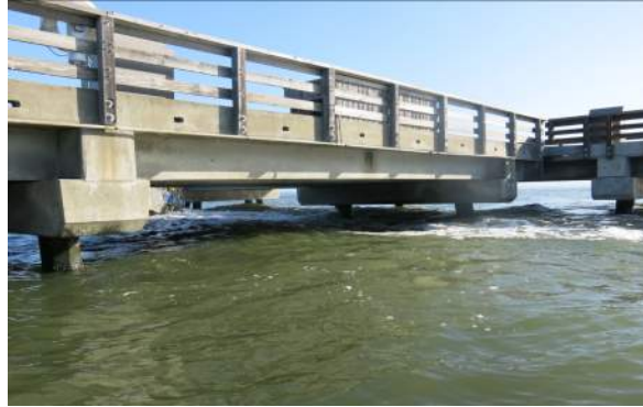
Photograph 16: Span 13-14 south face
