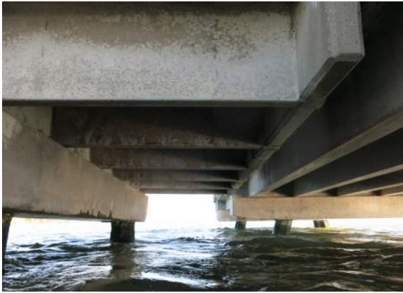
Photograph 15: East end of causeway (at exp. jt.)
