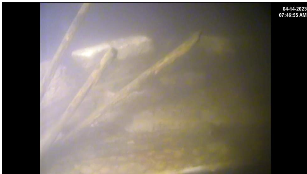
Photo 2 – F14 – North Face – 10 feet below surface – Vessel debris abutted to pile
