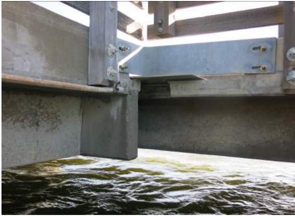
Photograph 17: Expansion joint - north side
