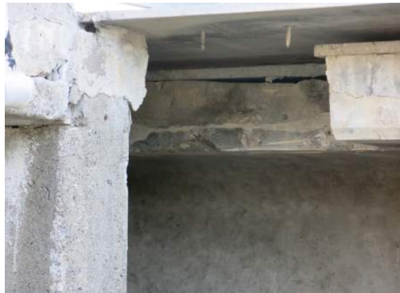
Photograph 19: Expansion joint - south side - detail
