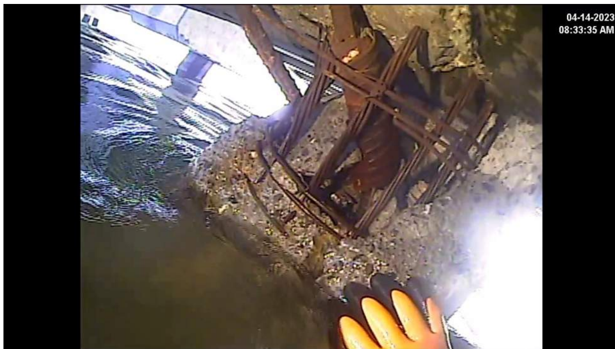
Photo 8 – F14 – North Face – Top of pile showing severe damage
