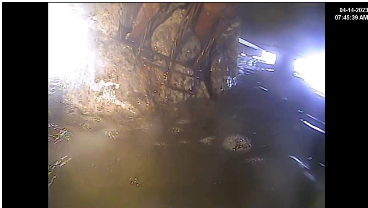
Photo 1 – F14 – North Face – Top of pile showing severe damage
