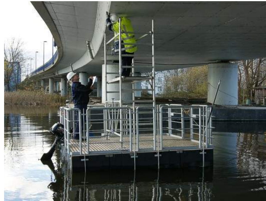
FLOATING WORK PLATFORMS
