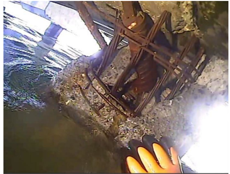
North Face – Top of pile showing severe damage
