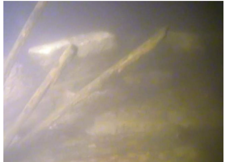
North Face – Top of pile showing severe damage
