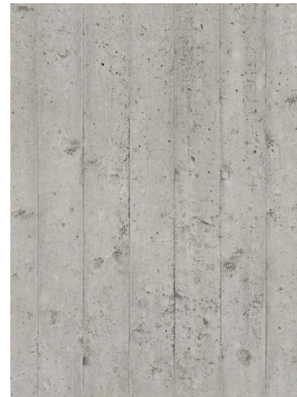
VERTICAL BOARD-FORM CONCRETE WALLS
