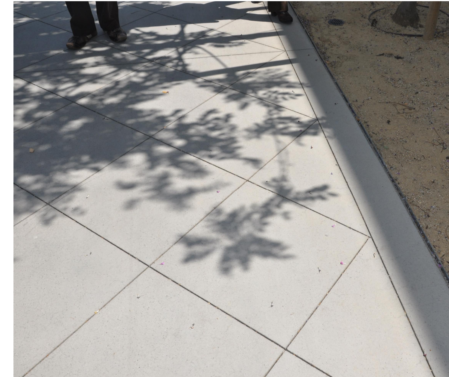
SAW-CUT CONCRETE PAVING
