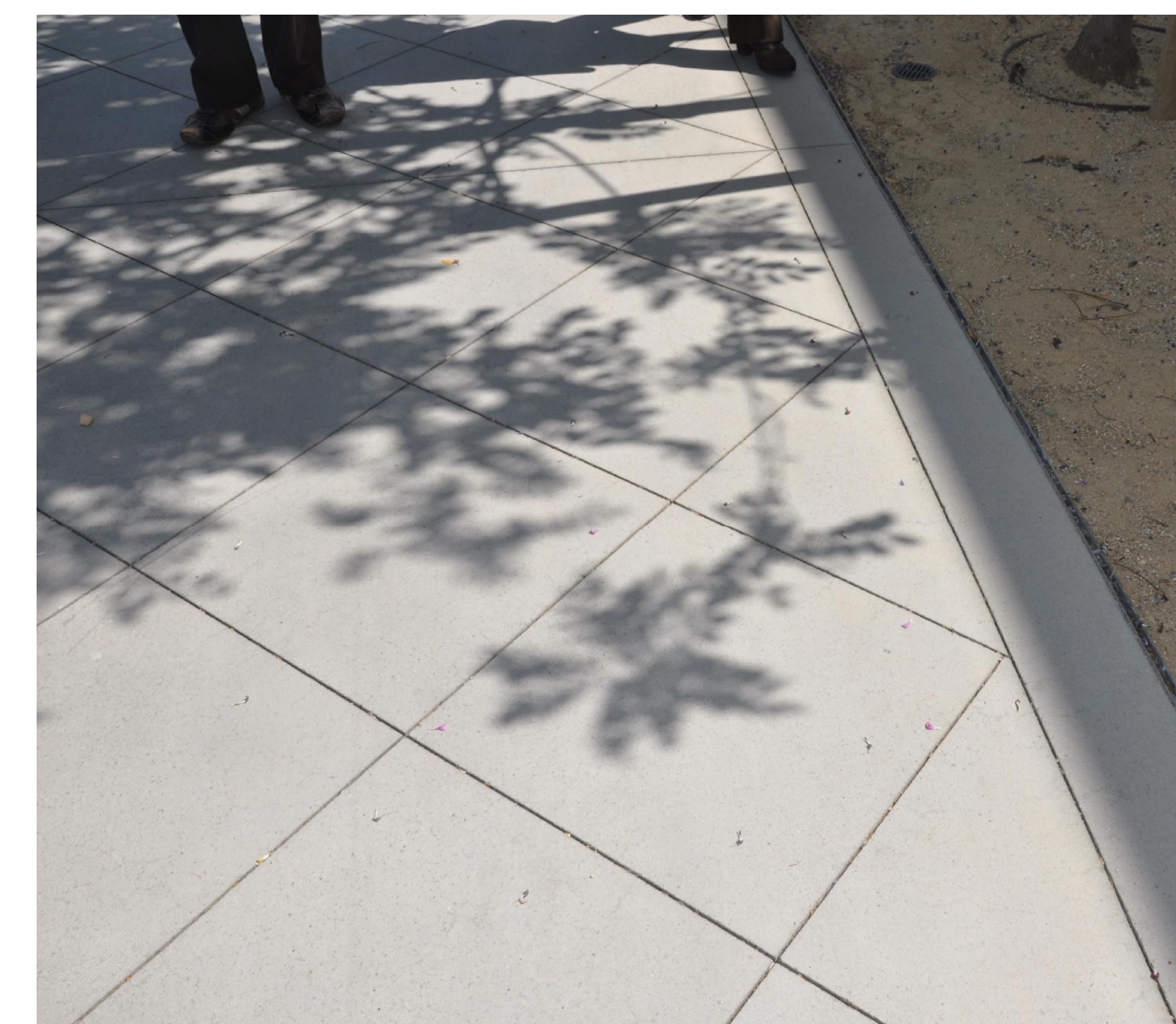
SAW-CUT CONCRETE PAVING
