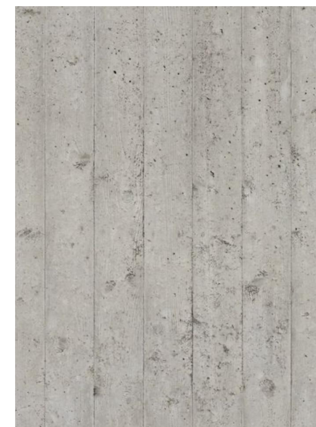
VERTICAL BOARD-FORM CONCRETE WALLS
