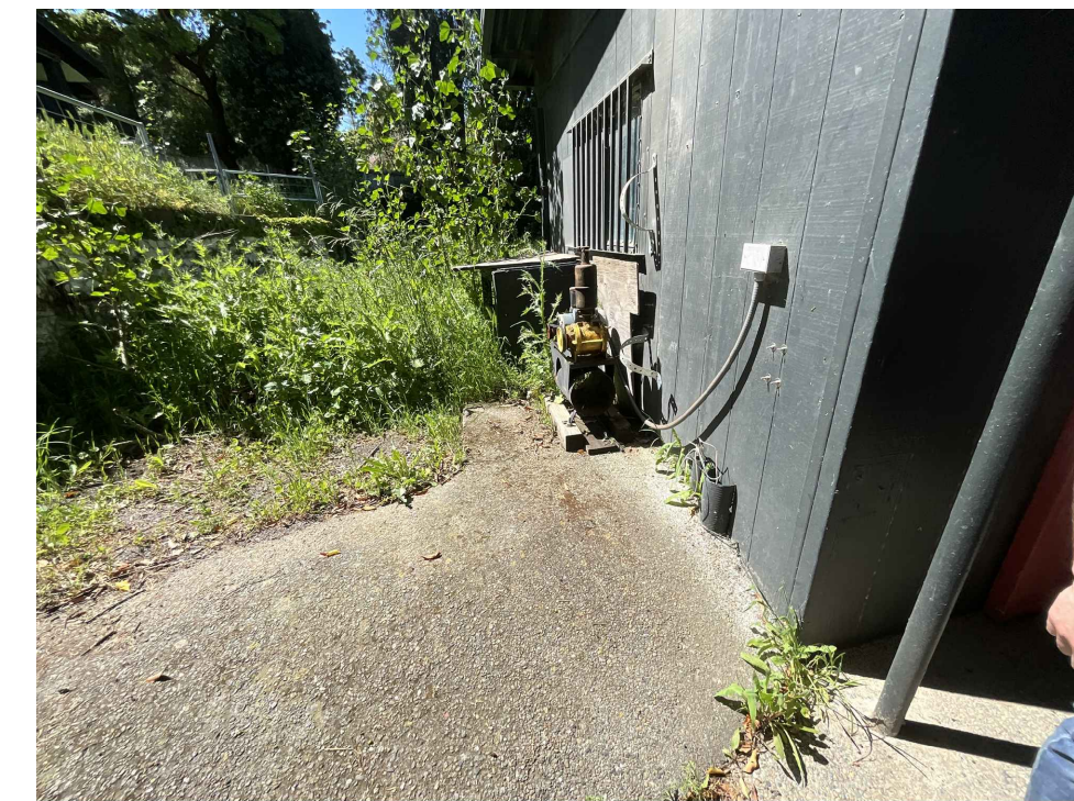
9 VIEW OF STORAGE UNITS FROM SIDE YARD
