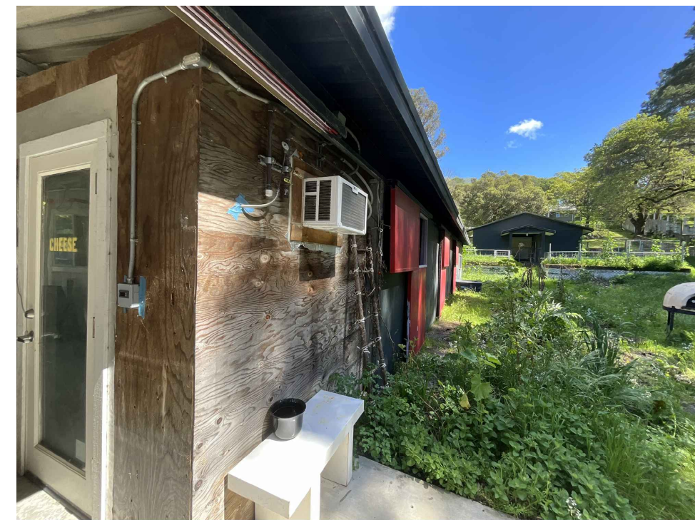
8 VIEW OF STORAGE UNITS FROM FROM REAR YARD
