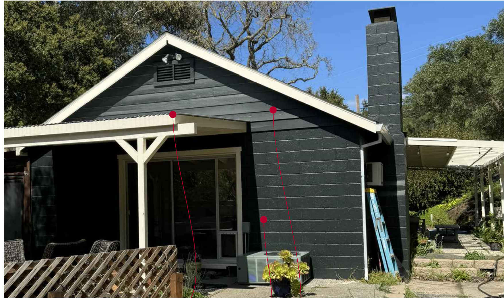
MAIN HOUSE ROOF: METAL TRIM/FASCIA: SMOOTH TRIM BOARD CMU: TROUPELLED FINISH COLOR: DARK GREEN/GREY HARDPLANK: VERTICAL SIDING COLOR: DARK GREEN/GREY DOOR & WINDOW:
