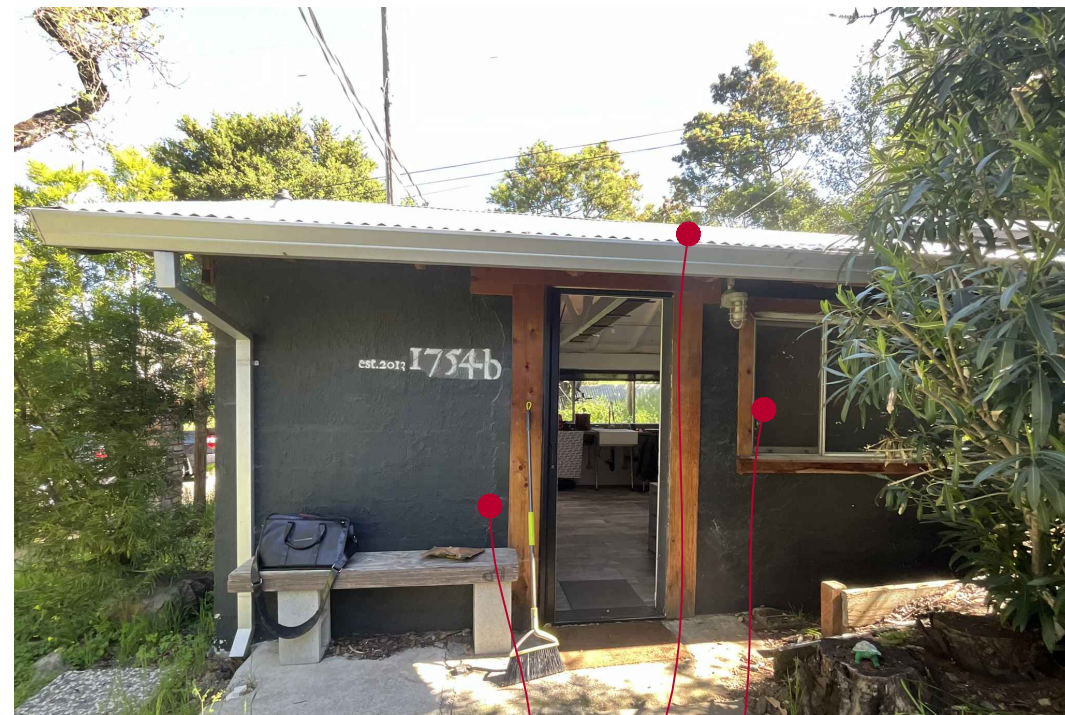
GUEST HOUSE EXTERIOR WALL: ROUGH STUCCO FINISH COLOR: LIGHT GREY ROOF: METAL DOOR & WINDOW: ALUMINUM
