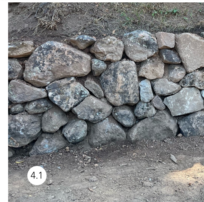
4.1 STACKED STONE RETAINING WALLS
