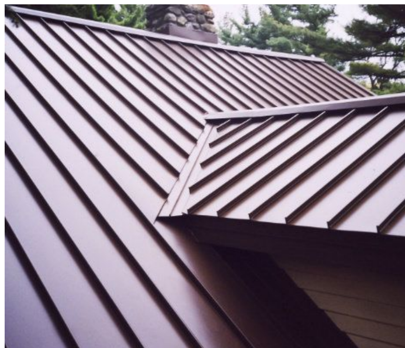
STANDING SEAM METAL ROOFING
