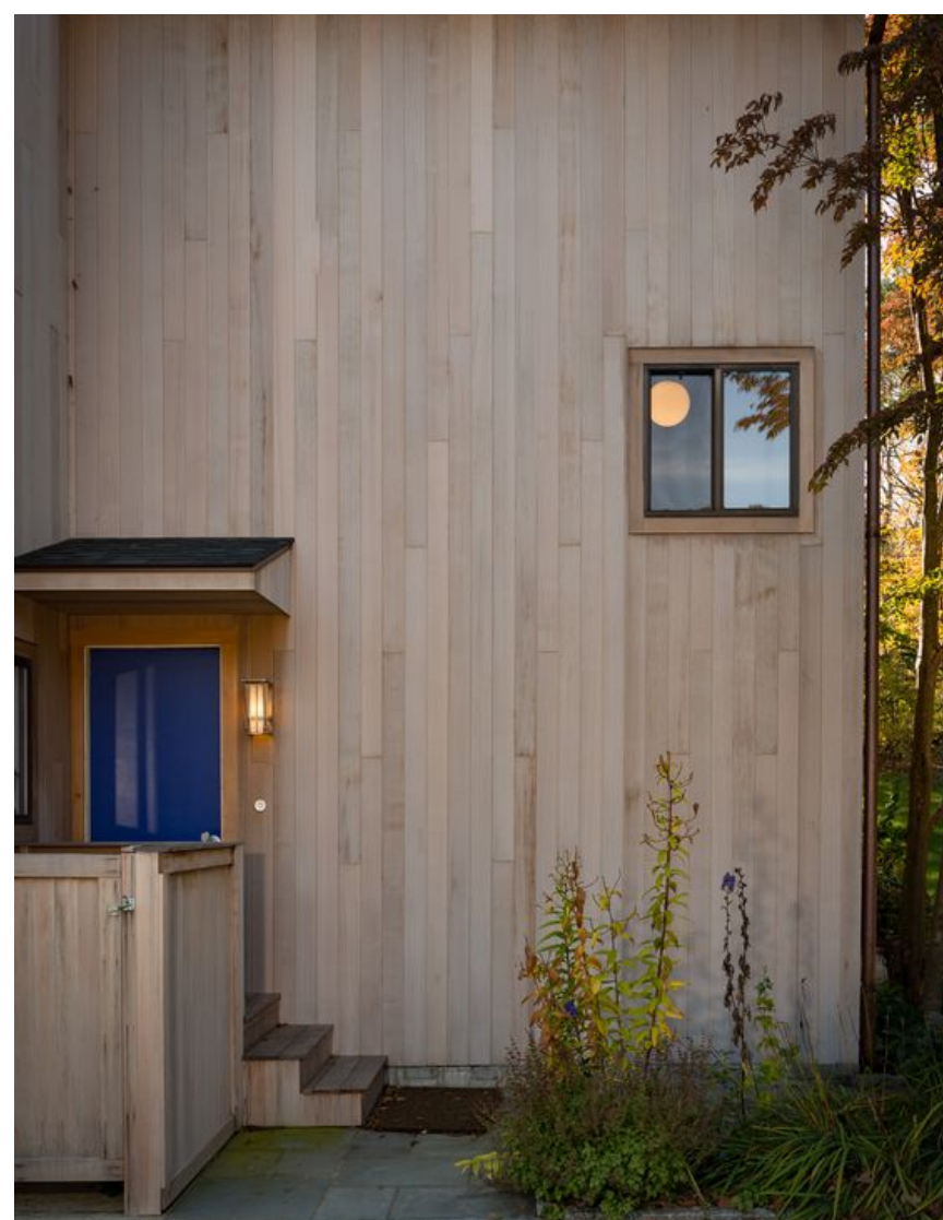
VERTICAL CEDAR SIDING & BRONZE WINDOWS
