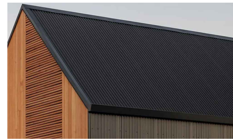
C ROOFING CORRUGATED METAL ROOF PANELS (7/8" RIB HEIGHT WITH 2.67" RIB SPACING) CLASS A FIRE RESISTANCE RATING COLOR: CHARCOAL GRAY
