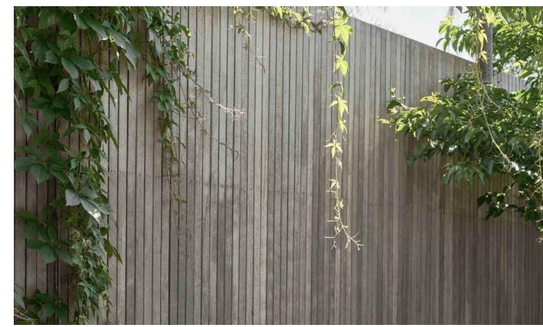
P WOOD FENCING THERMALLY-MODIFIED SPRUCE & PINE VERTICAL T&G WOOD BOARDS BY DELTA MILLWORKS COLOR: NATURAL GRAY PATINA
