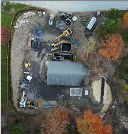
Between November and April, six AdvanTex AX-Max units were installed to replace Pinebrook's failed rotating biological contactor (RBC). The final photo on the right shows that the RBC and the building once housing it have been removed. (Photos courtesy of the Dutchess County Water and Wastewater Authority.)
